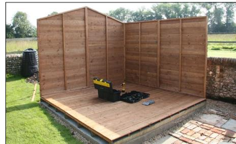
**4.** When all the side panels are screwed together walk round the shed and ensure that they are sitting squarely and evenly on the floor. Once you have done this, nail it through the battens on the bottom of the side sections into the floor. Use 3" nails on the apex end or pent end sections and nail into the floor battens. Use 2" nails on the sides.
