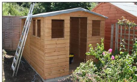
**7.** Nail the fascia boards (size 3"x1/2") on evenly with 2" nails. You will have 4 on apex sheds (2 for each end and which will need the angle cutting on them). On pent sheds you have 3 fascia boards. There is 1 on the high side of the shed and 1 to go on both ends.
